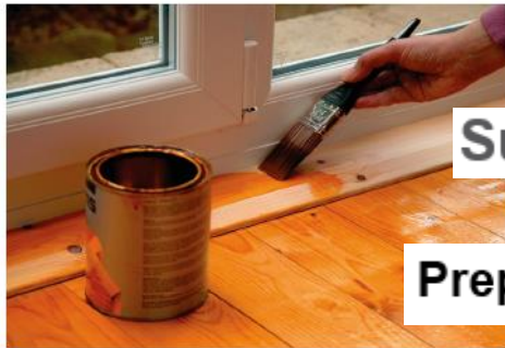
Figure 3.11.1 A cellulose varnish being applied to a softwood floor by hand. The varnish both accentuates the natural grain pattern and protects the timber from wear, increasing its durability.
